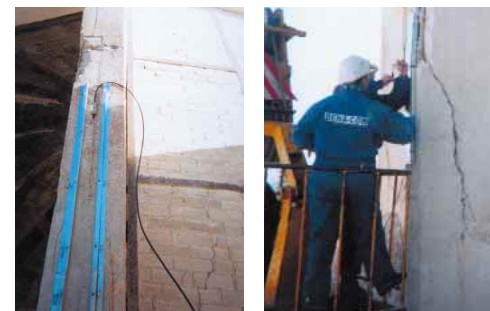
Placement of Osmos sensors on the dome's posts
