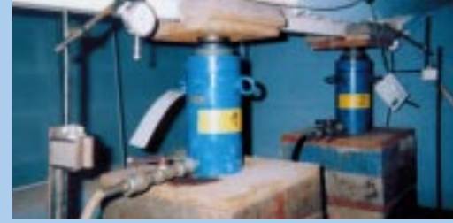
Hydraulic hoisting supports to shore up sagging
