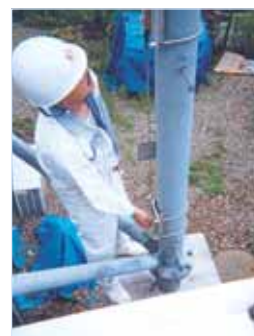
Installation of an optical extensometer by a JGC technician.
