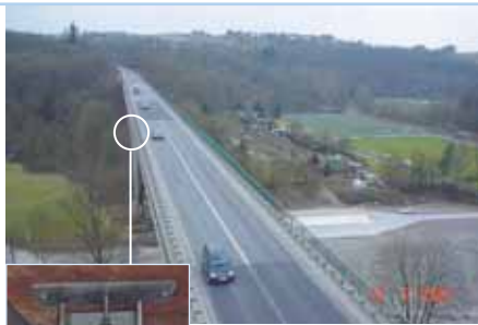
OSMOS-WIMS installed on the Viaduct of Murrthal (See p4) Above, one of the WIMS sensors.
