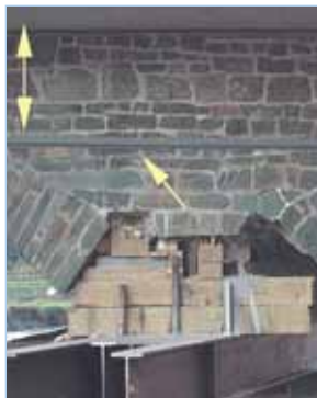
Emergency bridge shoring and optical strand in protective housing (see arrow).
