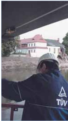
A TÜV technician installs an optical strand.
