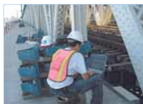
First in situ measurement and launch of the system.
