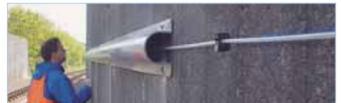
Optical strand of 10 m length installed on a curve section.
