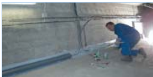
Optical strand regulation prior to housing installation
