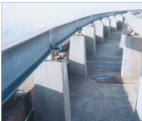
Gantry track, inside and outside rails
