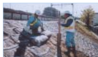
Control point coverage
