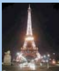
The OSMOS system operated in real-time on the Eiffel Tower since 10/27/1993.
