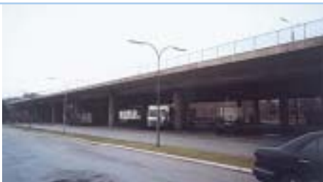
The Skovdiget bridge, near Copenhagen
