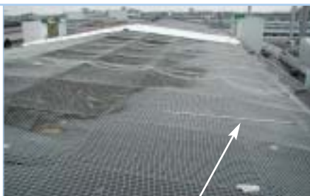
Protective net on roof; optical strand installed on brace
