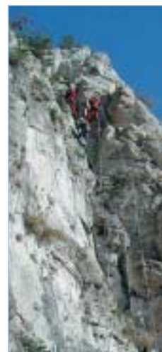
Climbers at work during the installation
