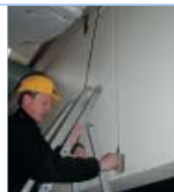
Installation of an optical strand
