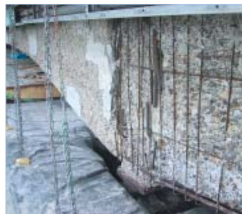
Scraping of a zone prior to repairs
