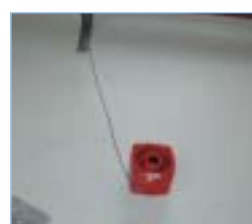
Warning siren connected directly...
