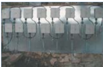
Battery of 15 X-Triggers connected to the 3 «harps»
