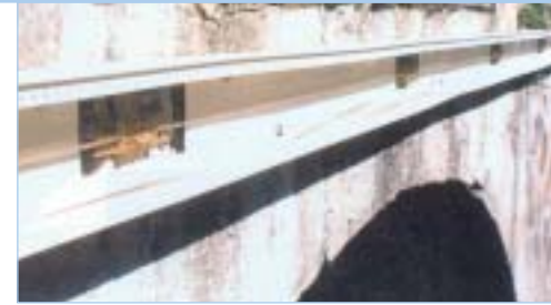
7 meter optical strand on the tympanum
