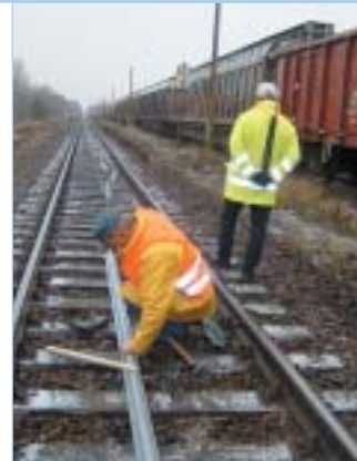
Installation of protective housing on the optical link network
