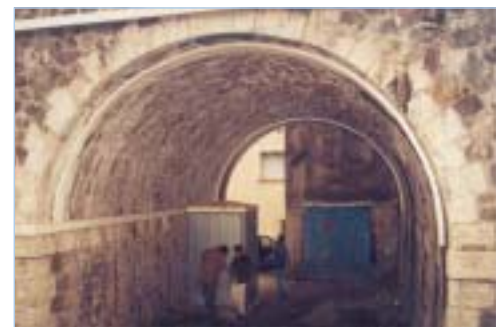
Installation of optical strands 8, 9, 10, and 11, 12 13 on the intrados of arch 28
