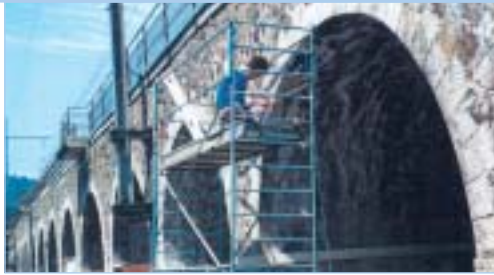
Installation of the optical strands, June 1994
