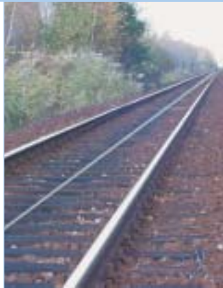
Optical strands positioned over a length of 800 m
