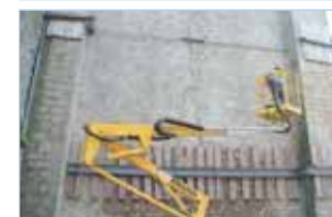
Installation in one day using an aerial basket
