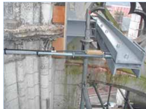
The LANFRY Company in charge of the restoration work has reinforced the nave using numerous tie-rods and wall-holding brackets that constitute a kind of corset to consolidate the edifice during the work
