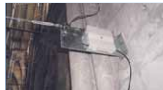
The LANFRY Company in charge of the restoration work has reinforced the nave using numerous tie-rods and wall-holding brackets that constitute a kind of corset to consolidate the edifice during the work
