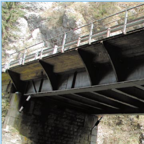
EX-Large measures between abutment and bridge.
