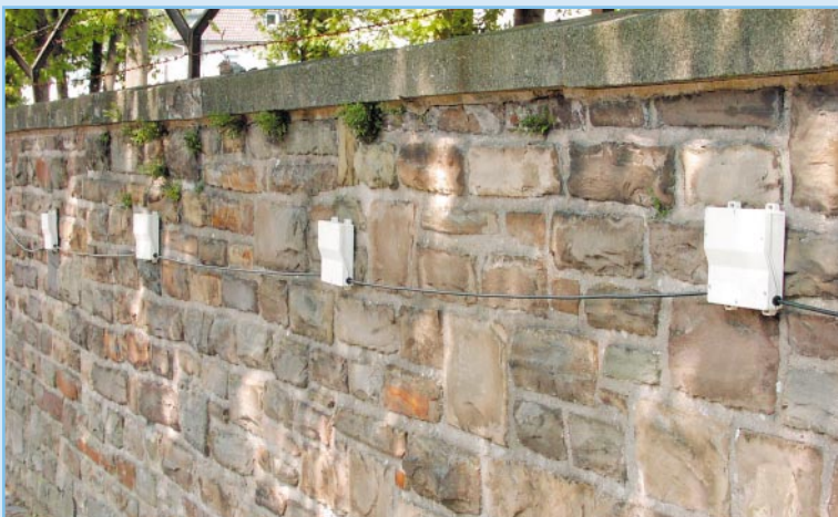
Wired X-Trigger on an extended wall.
