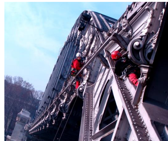
Installation team, fixing sensors under the viaduct
