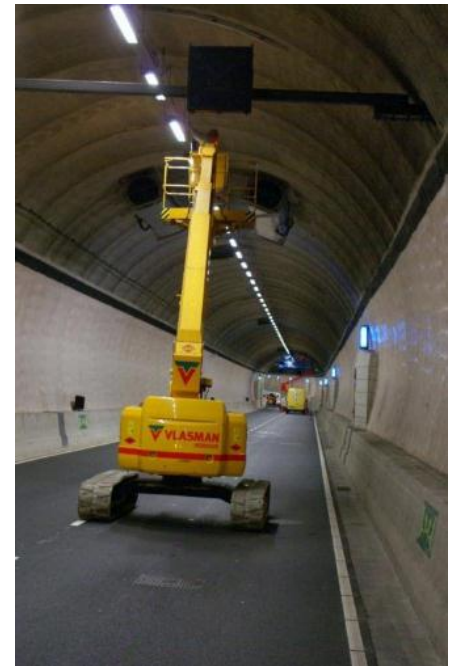
Aerial lift utilization to fix the Optical Strand in the tunnel
