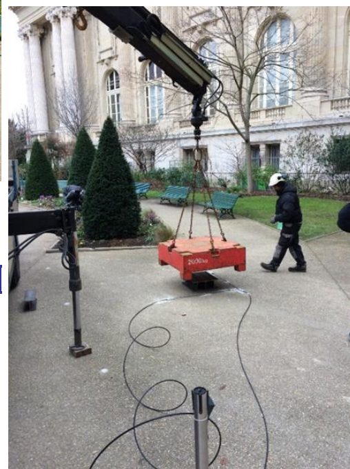
Static loading test with 2 ton loads
