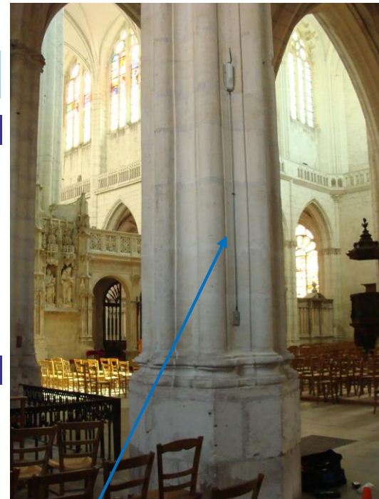
LIRIS Optical Strand on a nave pillar, before protection
